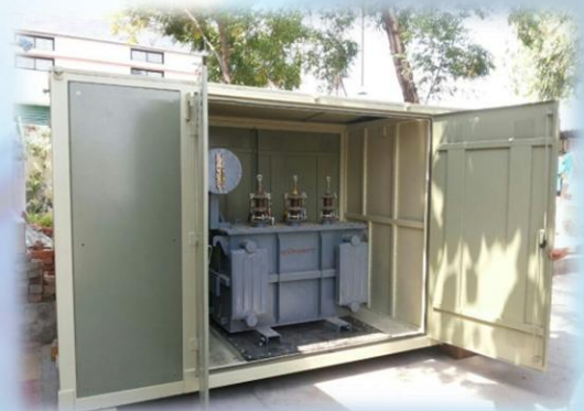
Compact Transformer Cubical
